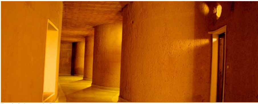
Earth Columns At Banasura
